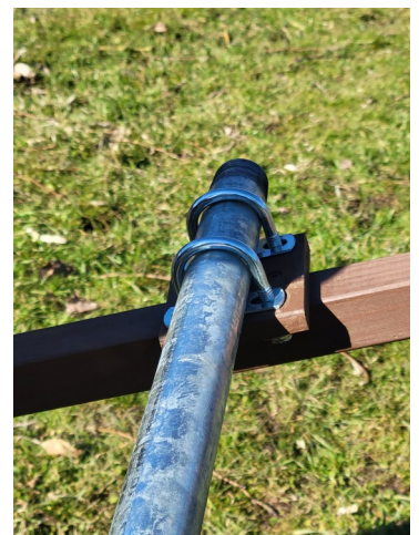
Mounting mechanism to mount raptor perches onto the pipe using U-bolts with stainless steel nylon locking nuts.
