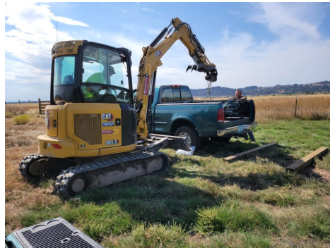
September 18-29. Mini excavator and crew arrive to lay out line, dig post holes and set posts in gravel, set wooden braces, lay out bottom barbed wire, place T-posts, and lay out woven wire.
