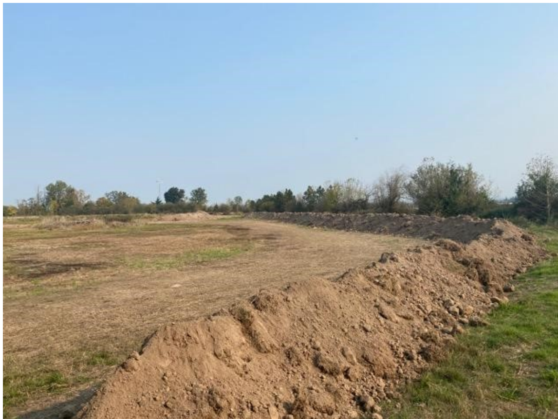
Dirt from old berm moved next to ditch area. Dirt will be used by SWCD to cover the ditch after the pipe has been installed. (Oct 2, 2020)
