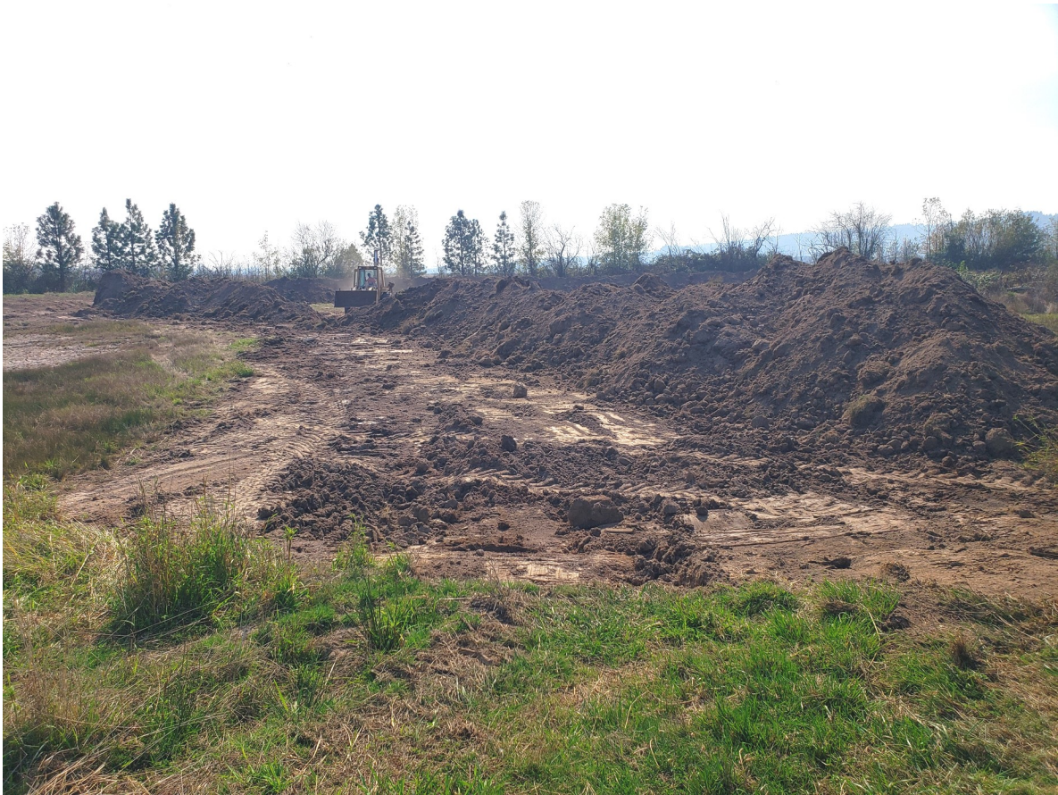
Old berm broken up with excavator. (October 2, 2020)
