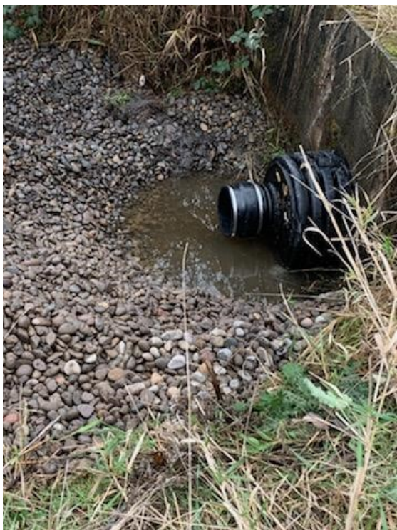
Reducer installed by SWCD. (Nov 16, 2020)
