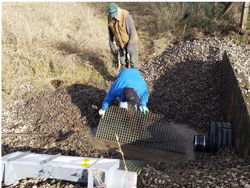
Installing base for flume. (Nov 19, 2020)
