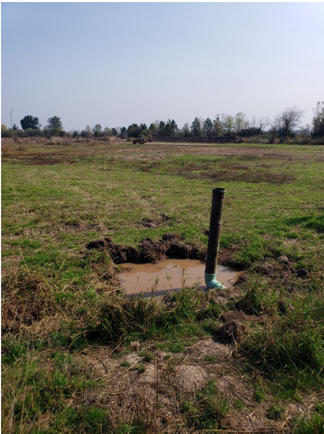
Installing pond overflow. (October 1, 2020)
