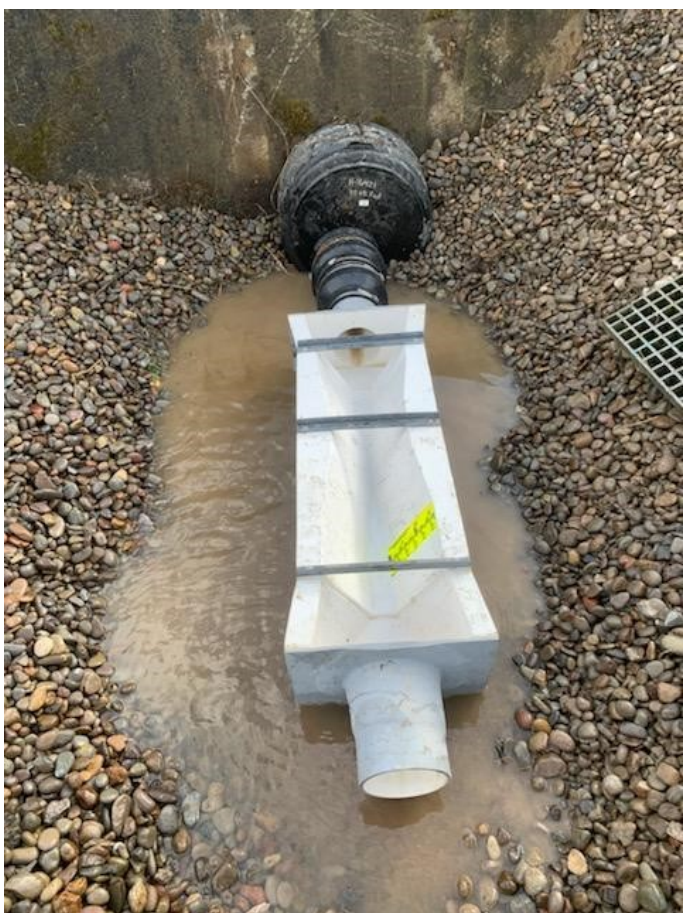
Flume installed. (Nov 19, 2020)
