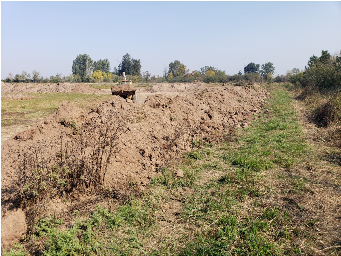
Dirt from the old berm moved to ditch site to be used to cover the ditch. (October 2, 2020)
